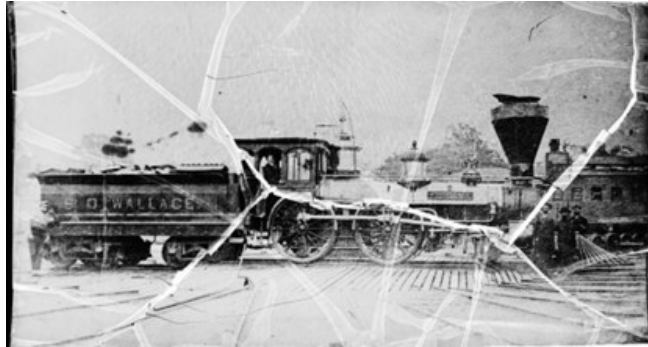
A fractured glass plate negative in the Steamtown National Historic Site collection shows Wilmington & Weldon's No. 36, a 4-4-0 built by Rogers in 1866. As a new superintendent takes the helm, Steamtown in Scranton, Pa., remains one of the most significant railroad preservation efforts on the continent, but its full potential has yet to be realized. National Park Service
