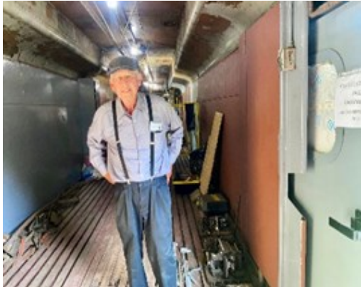
Volunteer Marco Zarate works on renovations in a 1918 Pullman baggage car at the North Carolina Railroad Museum. The museum has received a $280,216 federal grant to construct new exhibits, which will engage patrons with additional hands-on activities. The baggage car will be part of an exhibit detailing the roles of passenger and freight trains. NCRM
