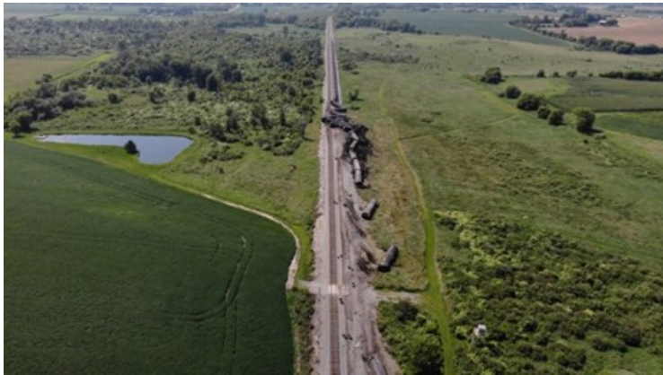
Approximately 22 cars of a 96-car CPKC unit crude oil train derailed near Reeseville, Wis., on Aug. 15, 2025. Dodge County Sheriff’s Office
