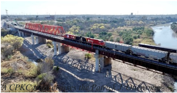
A CPKC train crosses the Patrick J. Ottensmeyer International Railway Bridge on Feb. 6, 2025. CPKC
