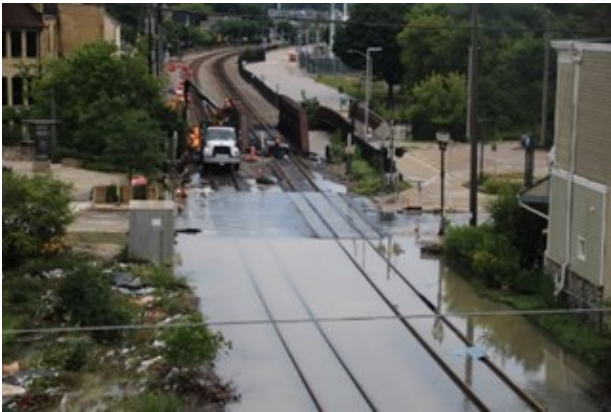
Crews work to clear debris at the CPKC bridge over the Menomonee River in Wauwatosa, Wis., where the tracks are under water after the river overflowed its banks. David Lassen
