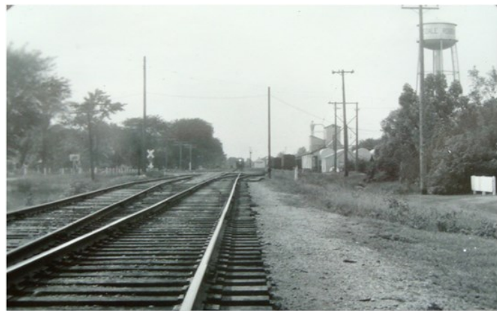
Looking north from 40-1/2 Ave. toward Noble Ave. crossing. Scars on the ties are from the recent change in the location of the track switch. Before World War II, the siding track joined the main line on the far side of Noble Ave. Late in the war the switch was moved to the south side of Noble and joined the main line where the scars are located. There were two more moves and a change in the angle of the switch before they were done. The final switch ended up located nearly at the 40th Ave. road crossing!
