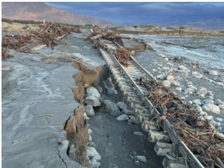
Flash flooding from Tropical Storm Hilary damaged Union Pacific's Yuma Subdivision in California in August. UP
