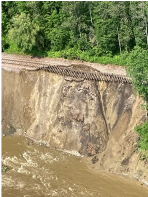
A slope failure on the Green Mountain Railroad at East Wallingford, Vt., is one of the areas where repairs continue as Vermont Rail System recovers from flooding earlier this month. Vermont Rail System
