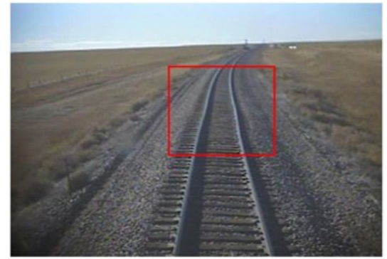
A still from the Empire Builder's in-cab camera shows a track defect that played a part in the train's derailment. NTSB
