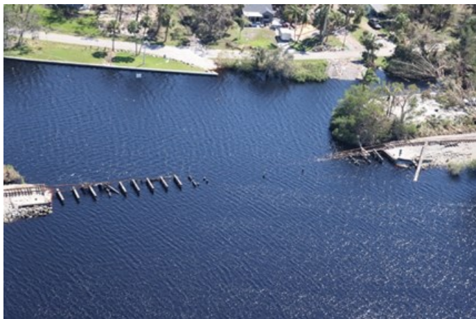
A view of one of six Seminole Gulf Railway bridges destroyed by Hurricane Ian. Sol Tucker
