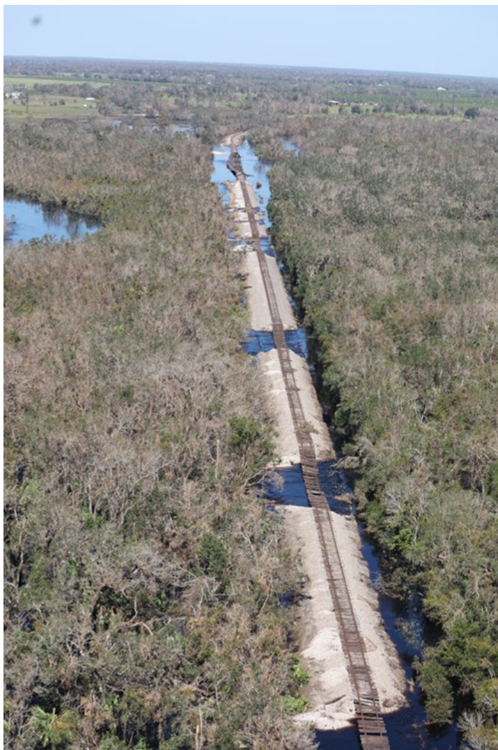
Multiple washouts scar a short section of the Seminole Gulf right-of-way. Sol Tucker
