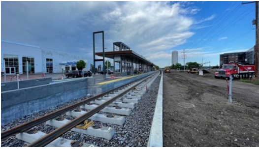
A view of the first LRT tracks being installed near the Downtown Hopkins Station.
