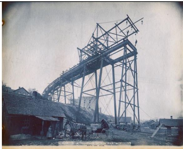
Erection of Iron Pier #11 Nov 17 1885
