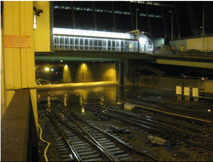
Above: Penn Station throat showing inflatable dam. More pictures in electronic edition extra pages. Photos from New Jersey Transit
