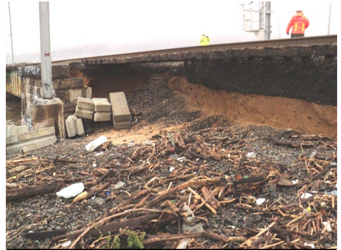
Washout at Perth Amboy. Damage photos from New Jersey Transit
