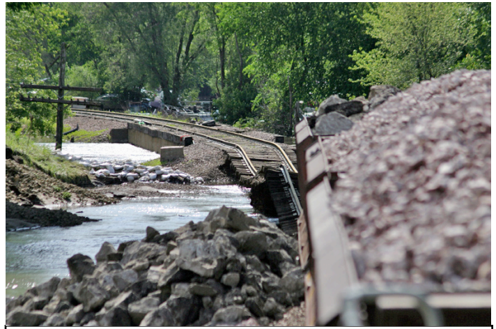
A Canadian National ballast train assists in repairing a washout west of Waterloo, Iowa, last week. Most of CN's Iowa Division is back up and running following devastating floods. Trains Newswire, June 17, Photo by Brian Root
