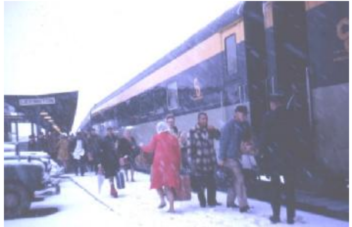
February 1969 - The eastbound Louisville section of the George Washington loads at the new Lexington Station. C&O passenger trains had been rerouted off a line passing through the middle of downtown to a belt line resulting in the relocation of the station to the east side of town. Photo by Russ Isbrandt
